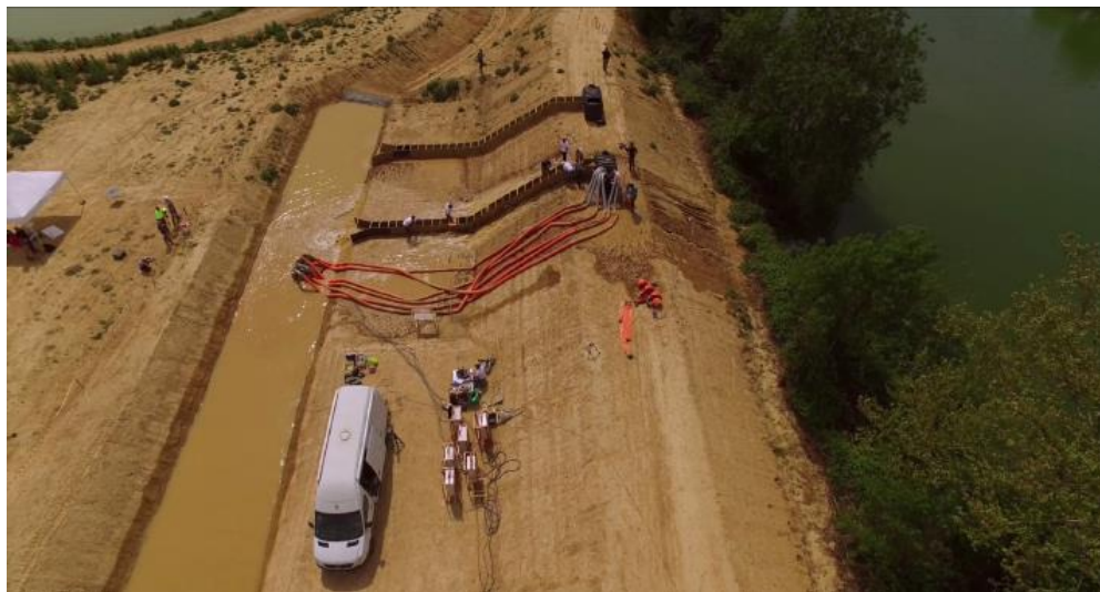
Figure 24: Overflowing tests on DigueELITE experimental dike (Bonelli et al. , 2019)
