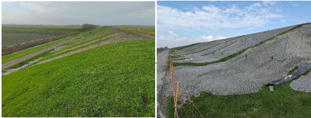
Figure 9 The results of covering the dike with saltwater sludge
