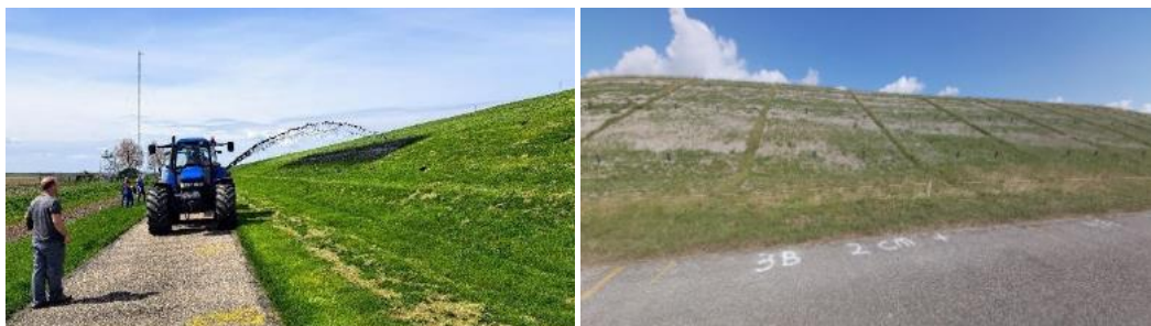
Figure 6 Spraying sludge and its result at the Westpolder in 2023
