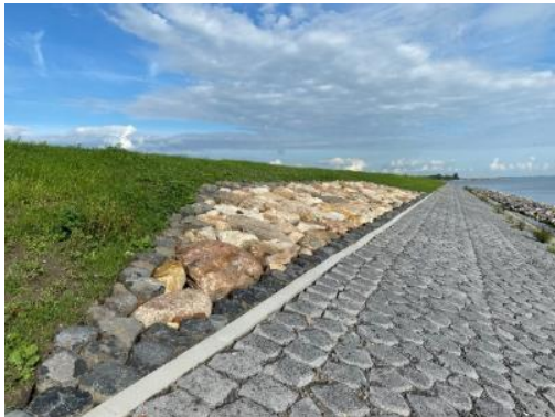
Figure 16: winter stay build into the new dike
