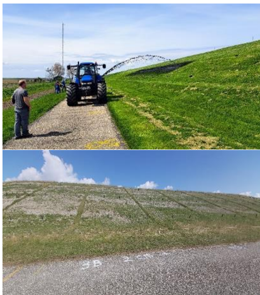
Figure 7 Spraying sludge and its result at the Westpolder in 2023
