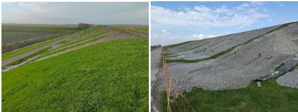
Figure 10 The results of oversurfacing the dike with saltwater sludge
